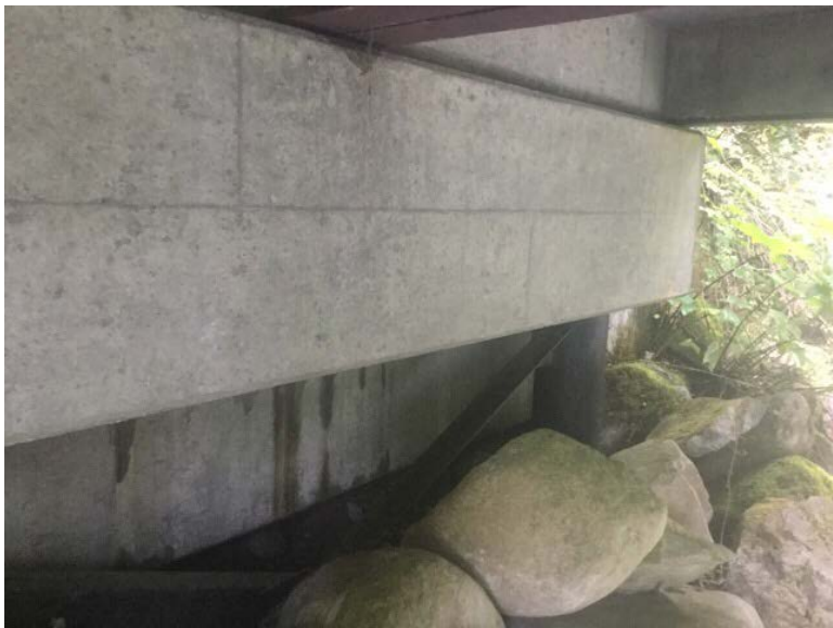
Right Bank Abutment when facing downstream
