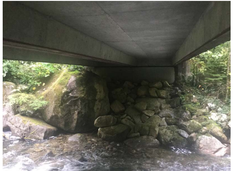
Left Bank Abutment when facing downstream
