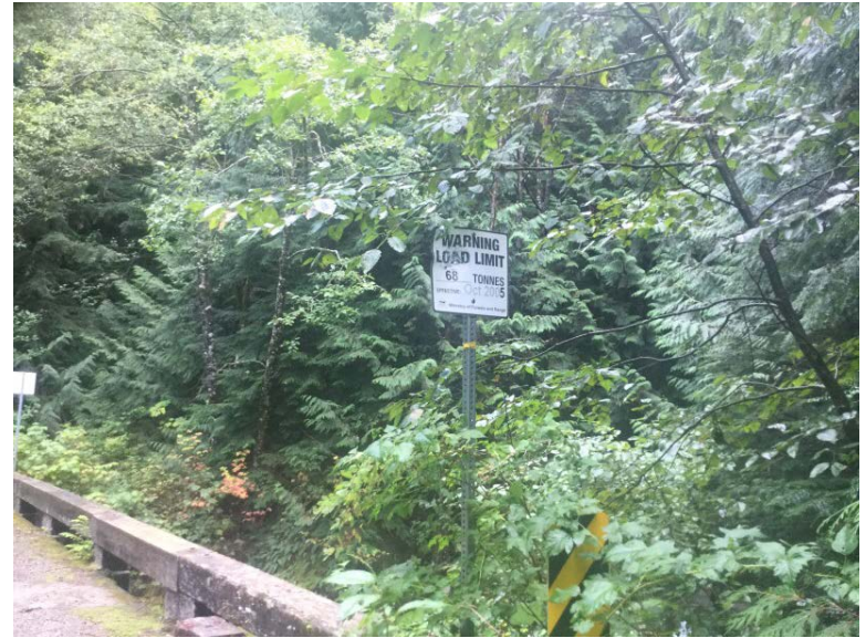
Load Rating Sign
